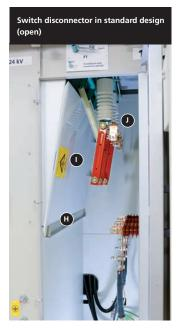
There is an opening at the bottom of the inner door directly below the handle that allows the door to be closed even when temporary earthing is connected.
